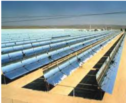
Parabolic Trough Concentrating Solar Collector at Kramer Junction, California Source: NREL 2012a
