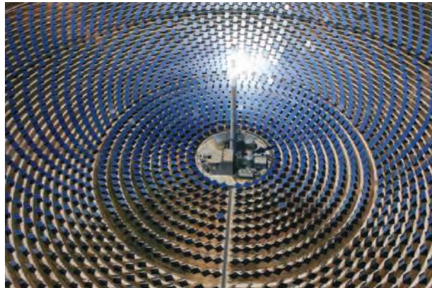
Gemasolar Solar Thermal Plant, owned by Torresol Energy ©SENER
