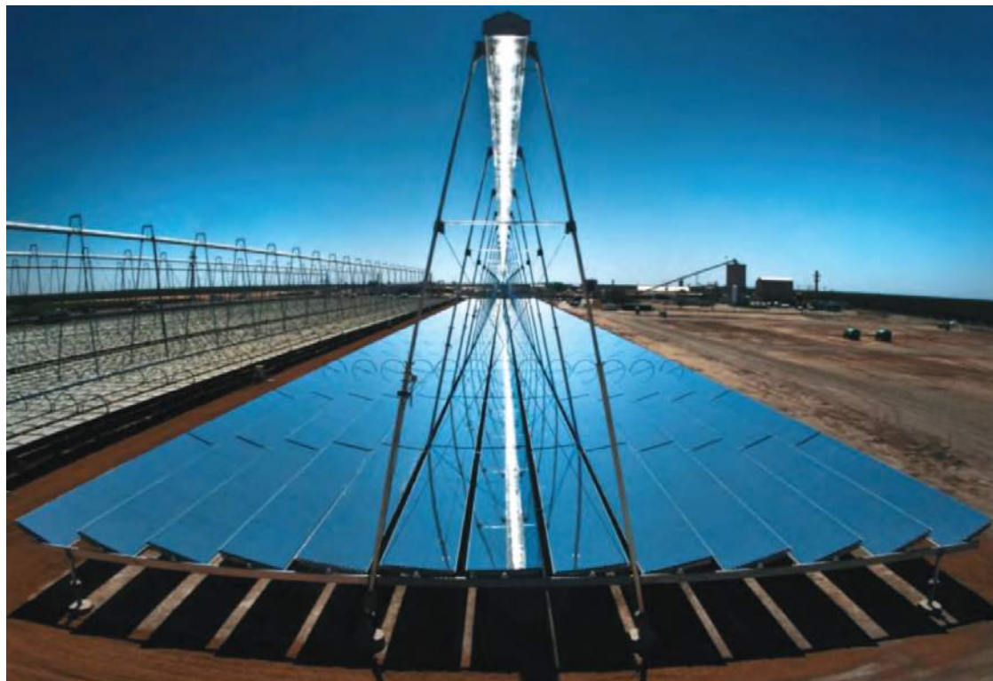
Figure 3.6 Linear Fresnel Collector Design 9
