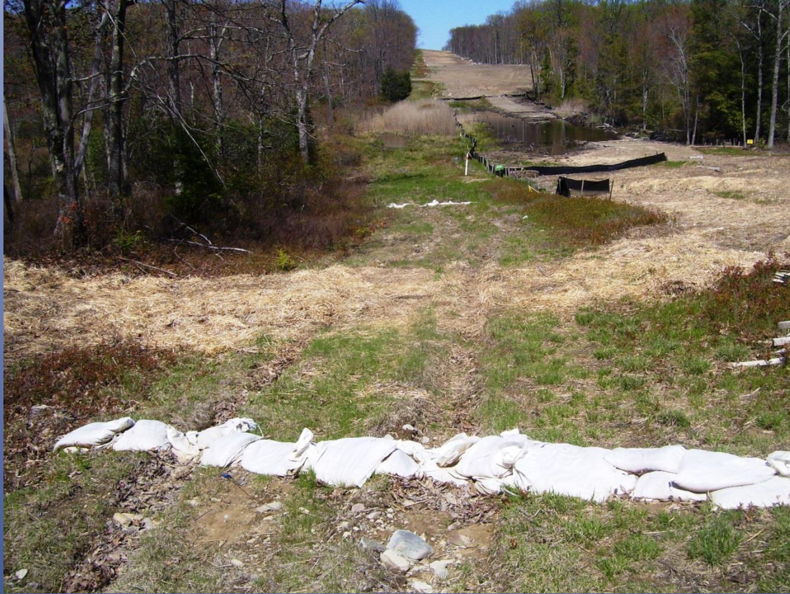
Sand bags used for erosion control
