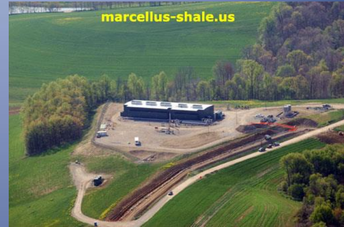
Photo of the Lowry Compressor Station , one of a new network of MarkWest compressor stations being constructed in Washington County, PA. These compressor stations often start out with one or two compressors, and shortly thereafter are expanded to four or five 1340 horsepower compressors that run on natural gas.
