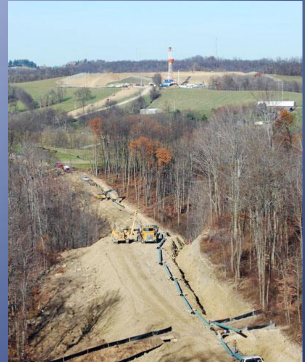
Amwell Township, Pennsylvania gas pipeline.
