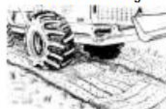
FIGURE 3.5 - Typical Tire Mat Wetland Crossing
