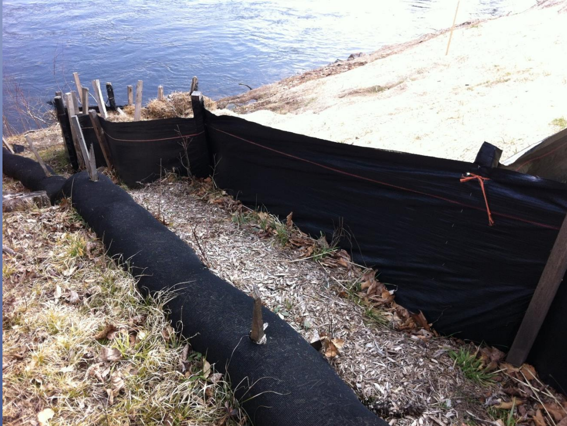
Perimeter Controls – Compost Filter Sock and Silt Fence
