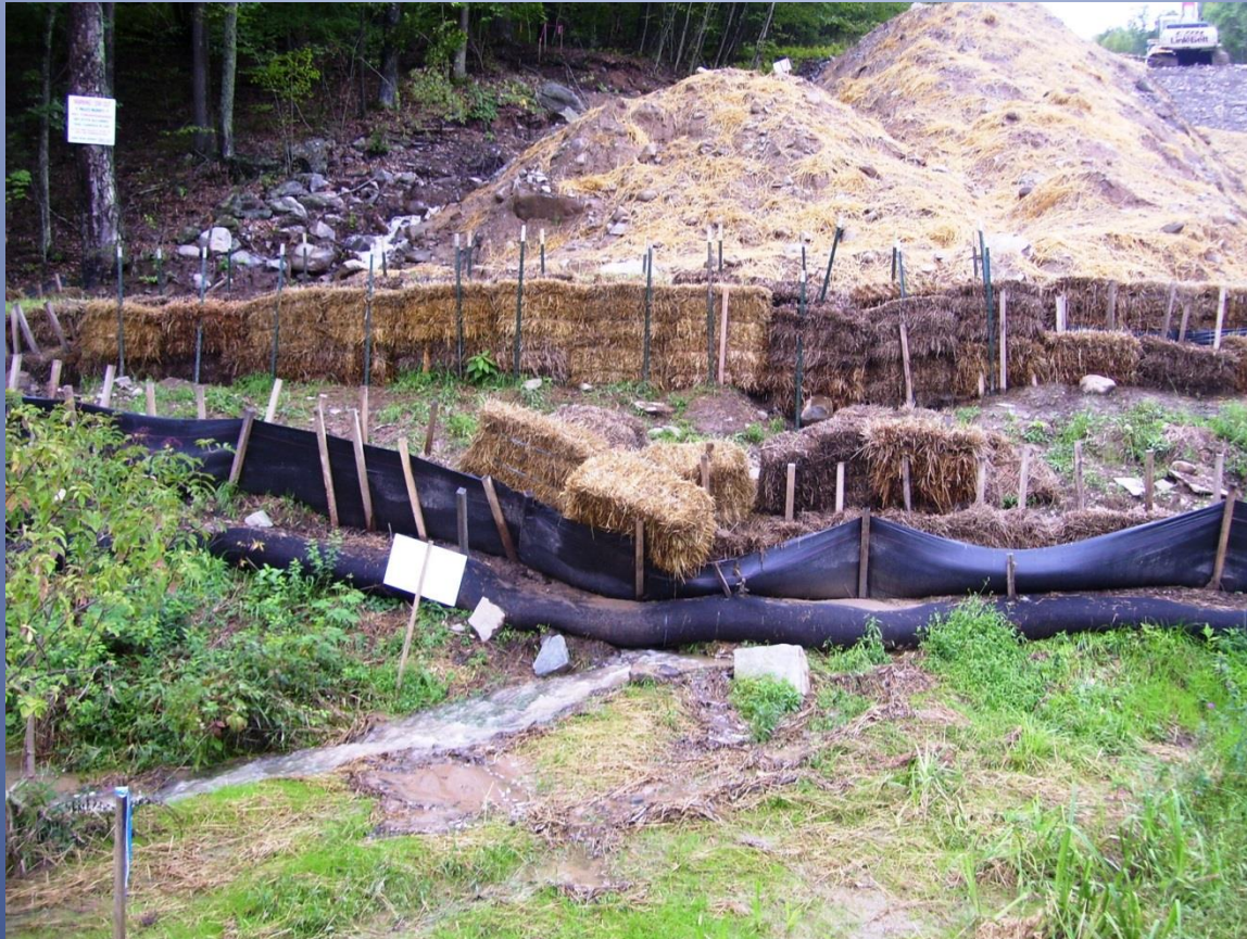
Top Soil Salvage and Storage
