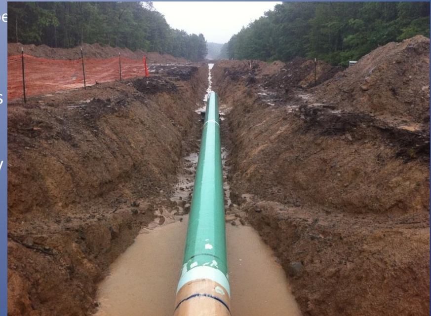
Tennessee Gas 300 upgrade line. Pike County, PA. 2011
