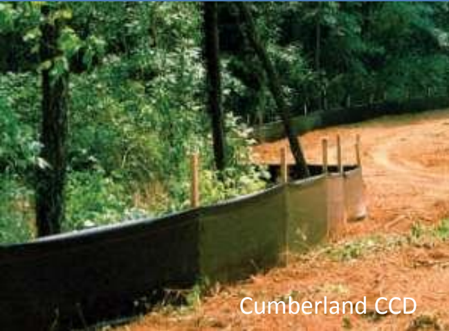
Silt fence – perimeter controls
