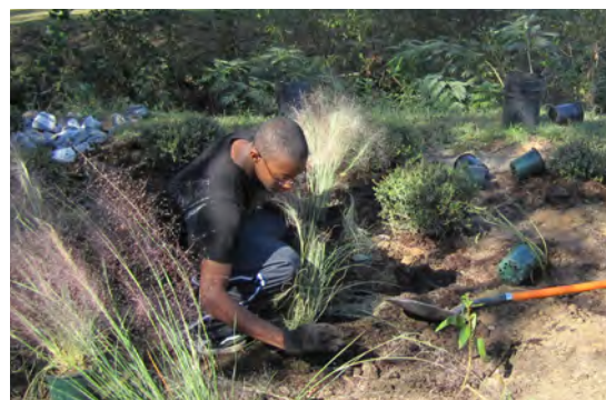
Rain Garden installation, City of Greenville
