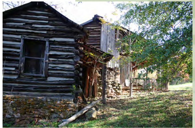
Vardy McBee's Brushy Creek Farm in Greenville, protected in 2010
