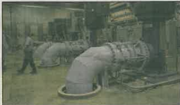
Water intakes on Lake Keowee draw 30 million gallons on an average day for the Greenville Water System. KEN OSBURN/STAFF
