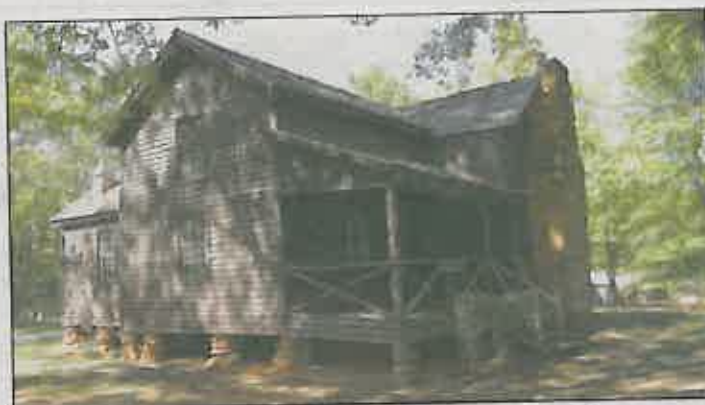
The Seay House is believed to be the oldest home in Spartanburg's city limits.
