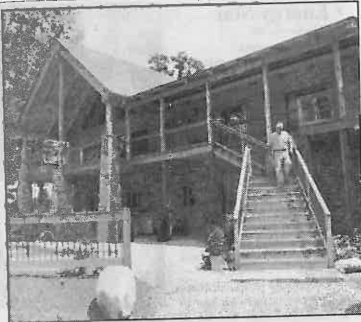
Schager, seen at his Energy Star log home in Gowan's Fort, will be giving a talk on energy efficiency concepts at a workshop tomorrow in Spartanburg. (photo by Jeff Byrd)
