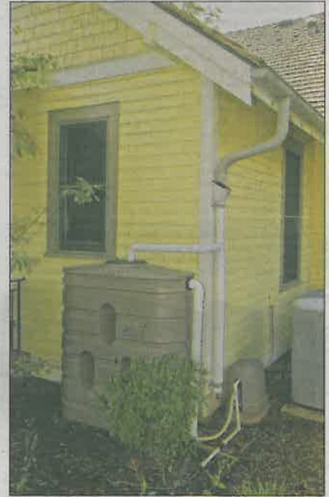
Piping will carry water from a rain barrel in the back of the property to other areas of the garden.
