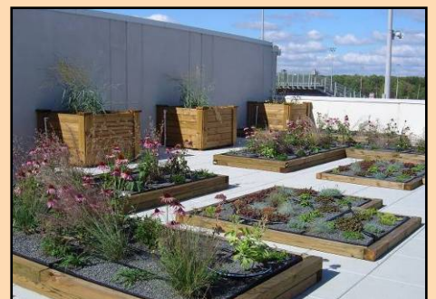
Intensive Green Roof on Riverside High School (Greer, SC)
