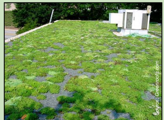
Furman Company green roof during establishment period
