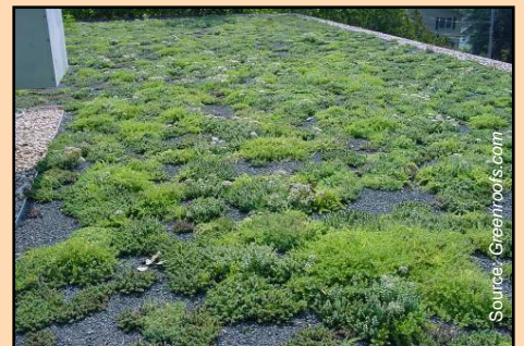
Extensive Green Roof on a Furman Company Office Building (Greenville, SC)
