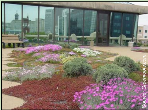
Intensive Green Roof Atlanta, Georgia, City Hall
