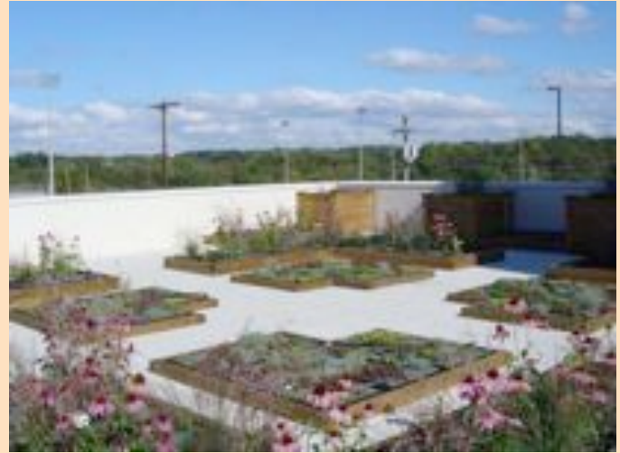
Mosses, sedums, lichens, and other drought-tolerant species are planted on the Riverside High School green roof in Greer, SC.
