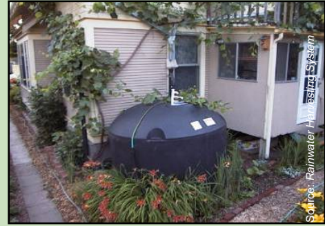
Residential Rain Cistern Portland, Oregon
